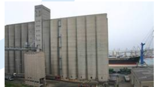
Silo conveying technique
